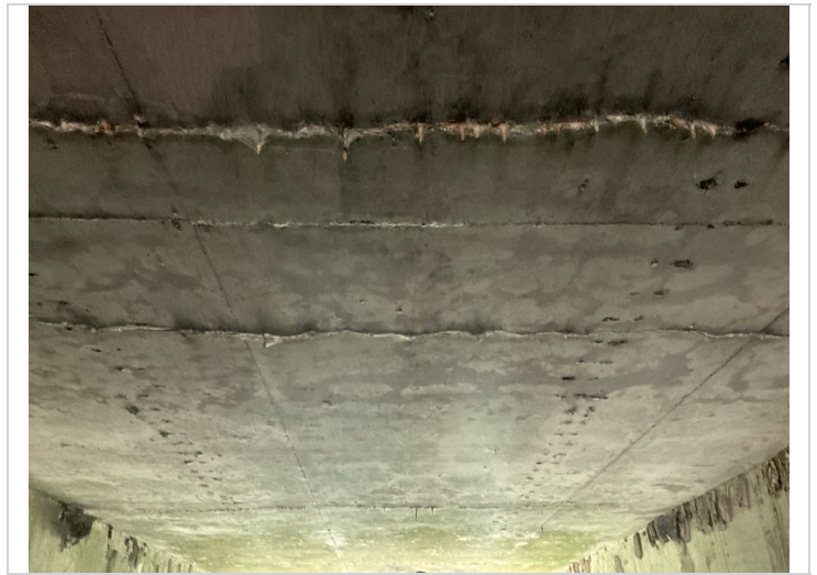
Cracks with efflorescence in top of barrel 2.
