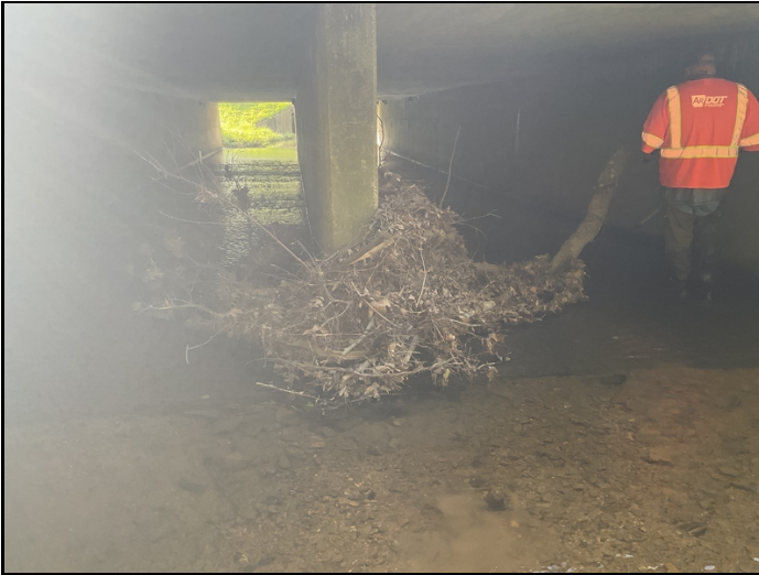
Logs and debris restricting water flow at inlet end of box culvert.
